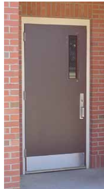
Ft Bragg Barracks Stairwell Door
